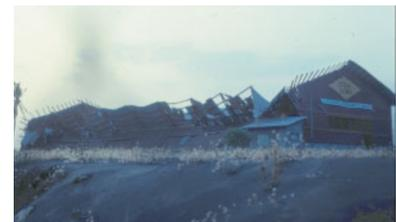
Figure 2: The mass load of a tephra deposit can cause building collapse.
